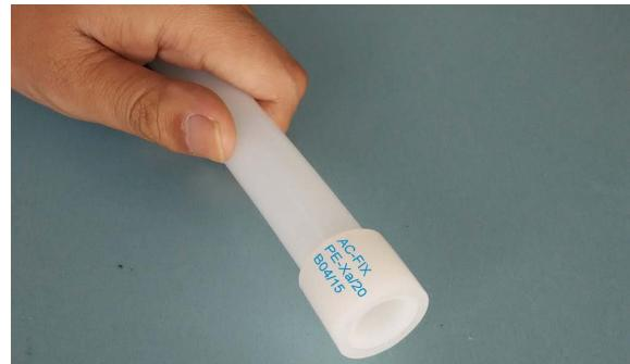
2. Fit the plastic ring into the pipe so that a very small part of it (max. 1mm) is outside the pipe end.
